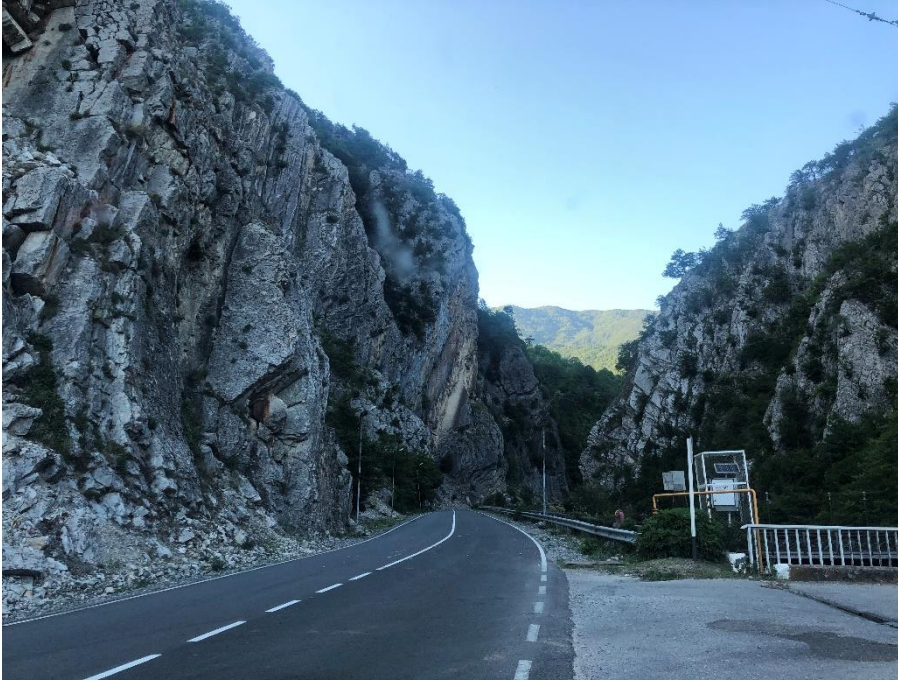
Pic.1 Proposed route near village Kvatskhuti, Ambrolauri Municipality.
